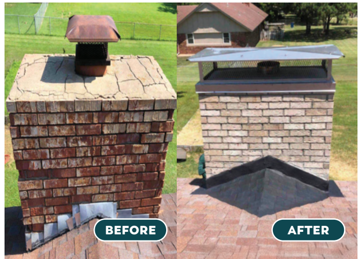
MASONRY REBUILD
