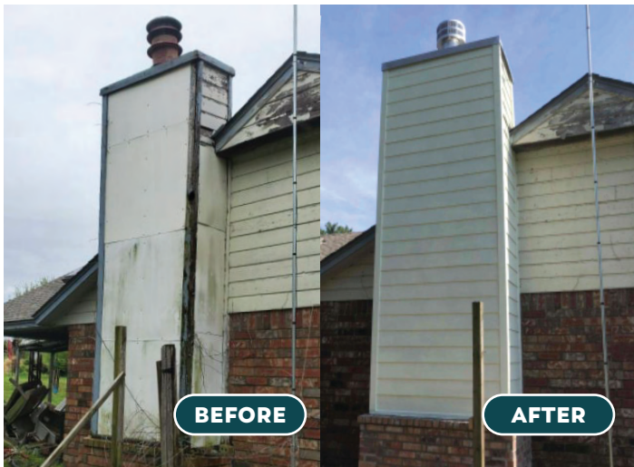
WOOD CHASE REBUILD
